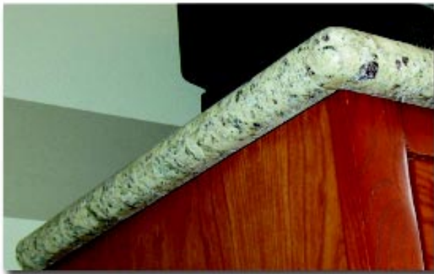
Saw cut marks are covered by the lip of the granite
